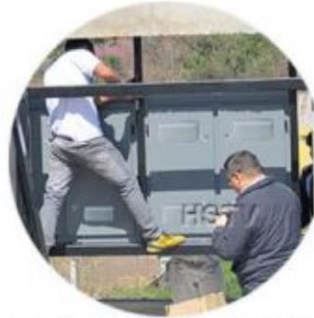
1. Installing led display to the steel structure
